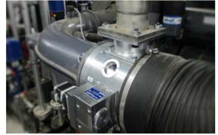
The VariFuel2-TEM air/gas mixer is based on the proven design of the VariFuel2 series and is specially designed for use with MWM® gas engines. Designed as a replacement and plug-and-play solution for the gas mixers used on the TCG 2016 series, the VariFuel2-TEM easily fits into the existing engine structure without any mechanical modifications.
